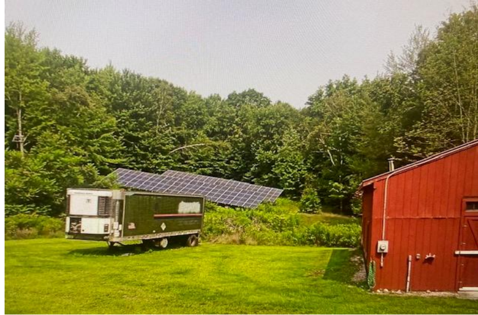
25kW residential solar array
