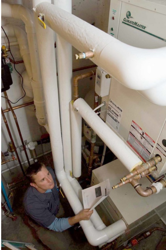
Worker adjusting the heat pump component of a geothermal heating system
